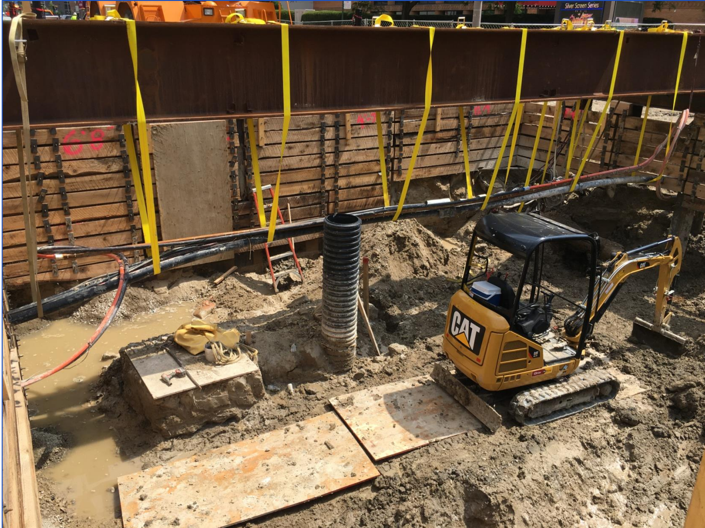
Adams / Superior Drop Shaft Construction
