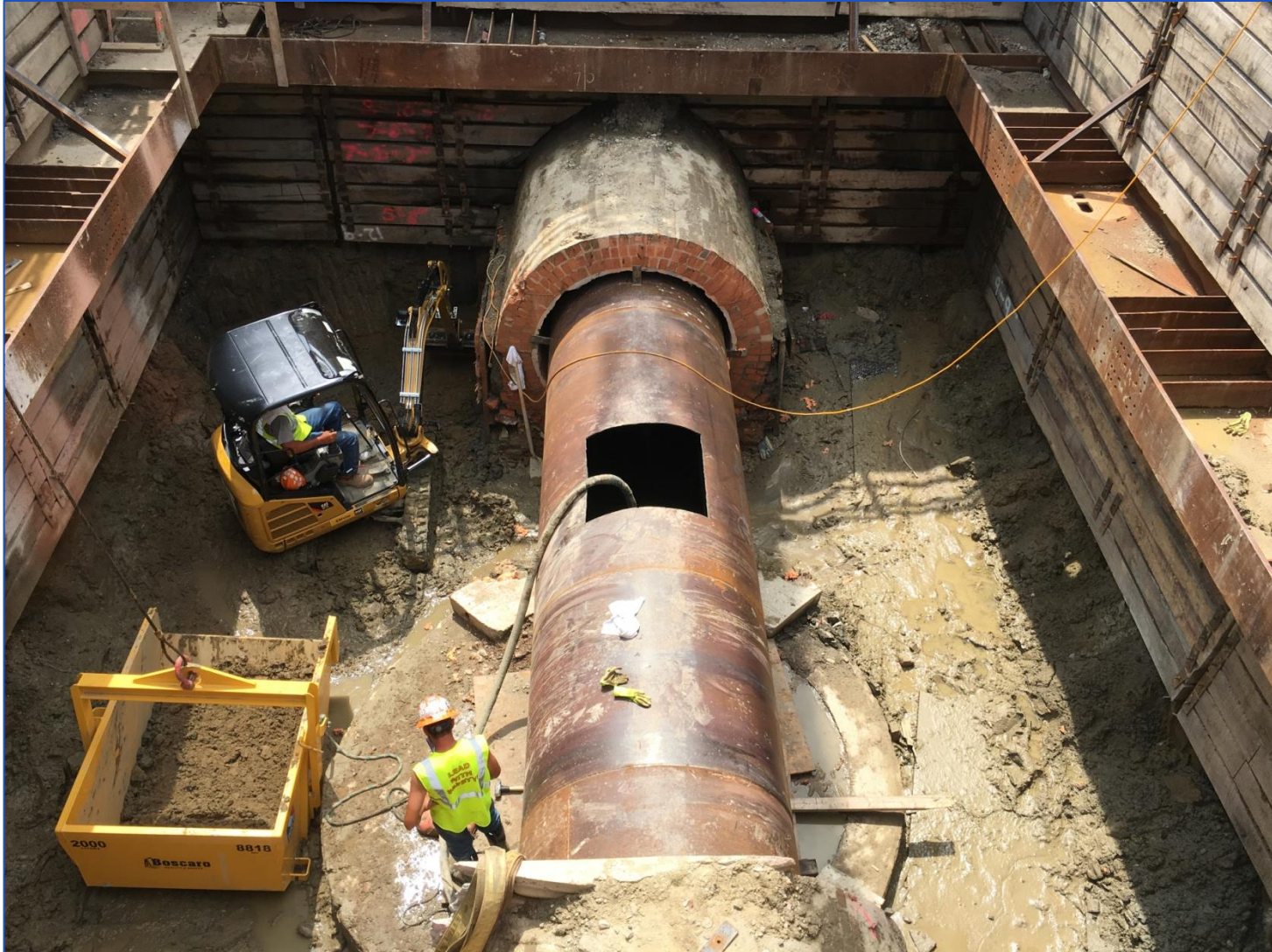
Orange / Superior Drop Shaft Construction
