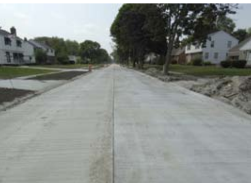
A new relief sewer under Beverly will help to eliminate sanitary sewer overflows in the River Road area.
