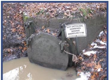
Not all pipes into the watershed are CSOs. In the photo above, a storm outfall on the left returns rain water to the watershed, and a CSO is on the right. Signage is used to identify CSO locations.
